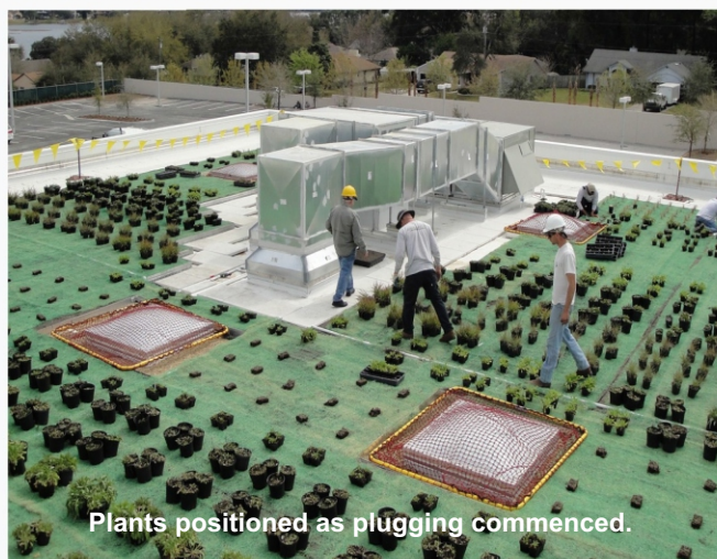
Roof protected by Curlex II QuickGRASS.
