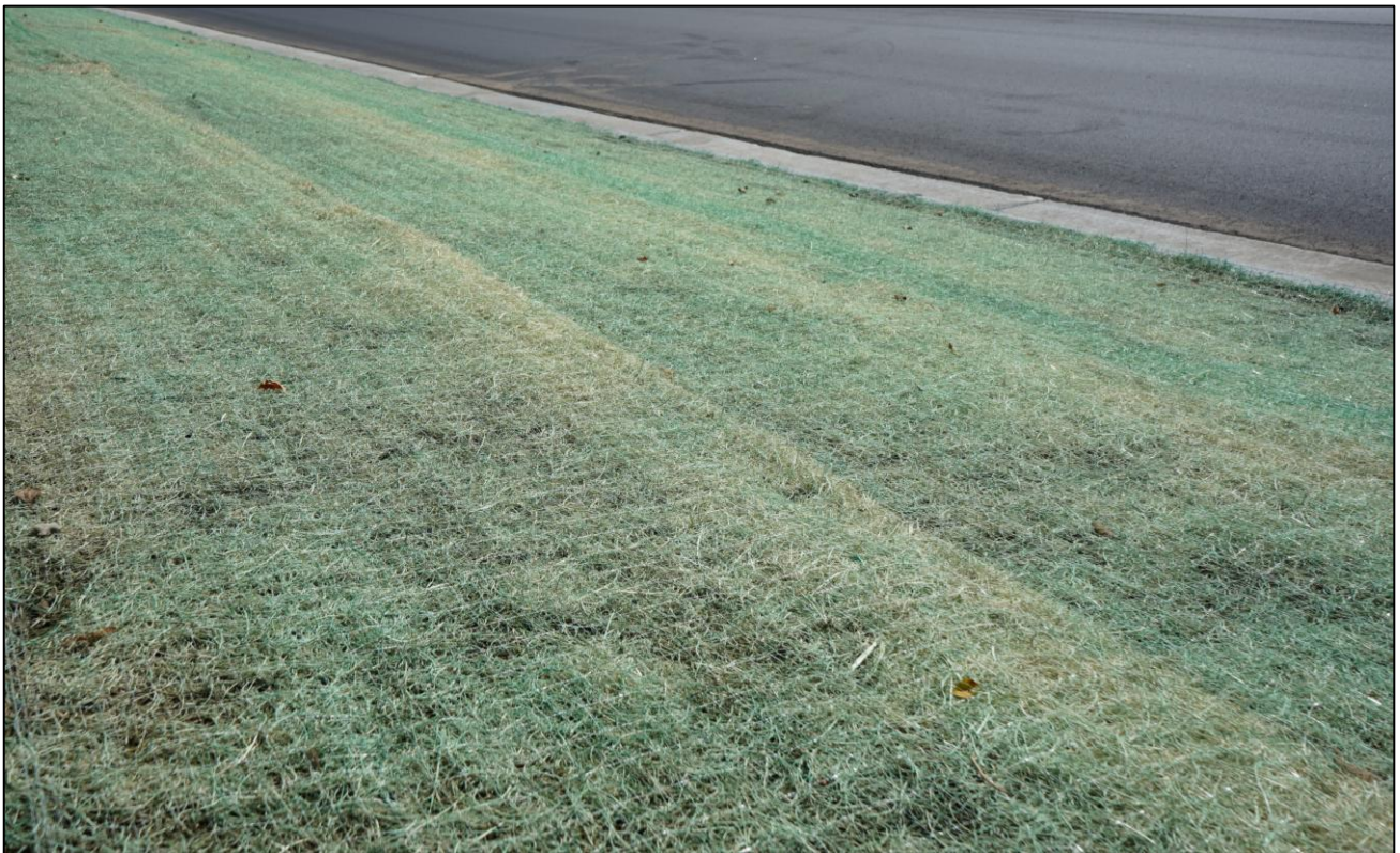
Figure 2: Curlex I QuickGRASS installed on a sloped roadside area.
