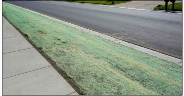
Figure 3: Curlex I QuickGRASS installed on top of the seed and soil amendments.
