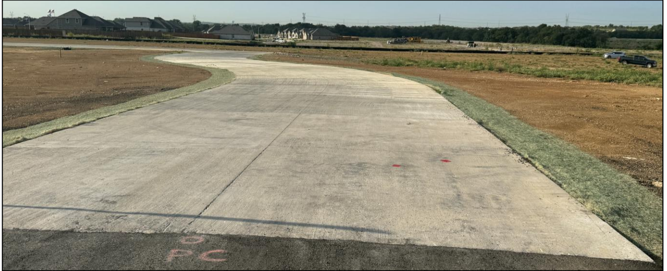
Figure 2: Curlex SiltTRAP installed on a street within the development.
