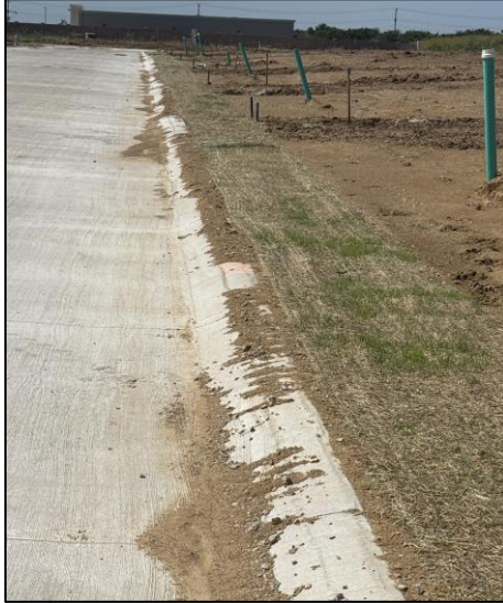
Figure 5: Failed straw buffer strip allowed sediment into the street approximately 14 days after installation.
