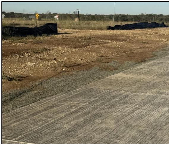
Figure 3: Curlex SiltTRAP installation where sediment was retained within the SiltTRAP and prevented from entering the street.
