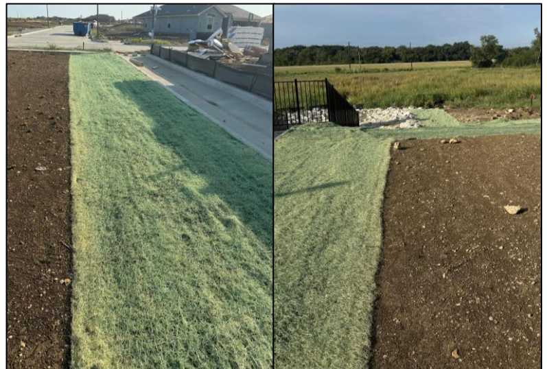
Figure 7: Recently installed Curlex SiltTRAP.
