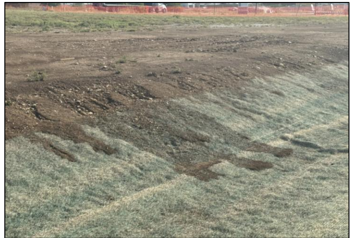
Figure 4: Curlex SiltTRAP installation that stopped flows of sediment.
