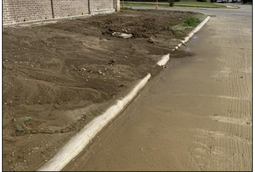
Figure 6: Failed straw buffer strip installation that was overrun by sediment-laden flows.
