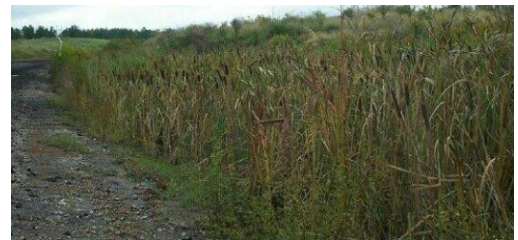
Roadside ditch bottom protected by vegetated Recyclex.
