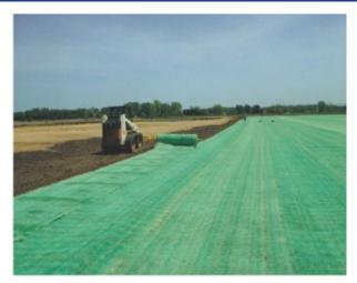
RoadRunner is a mechanically installed erosion control blanket system that has virtually rendered manual installation obsolete. If you work with large projects and would like to drastically reduce your unloading and installation labor rate, RoadRunner blankets along with our patented installation equipment is your most efficient solution.
