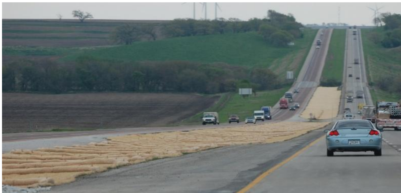
1. Curlex excelsior blanket and Curlex® Sediment Log® technology protecting water resources.
