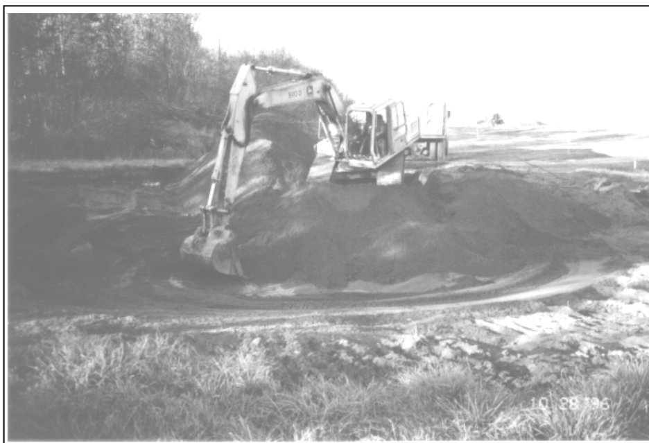
Figure 3. Excavation of ErosionLab's sedimentation basin, October, 1996.
