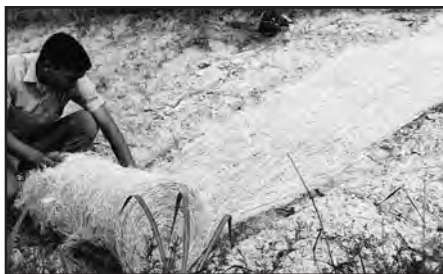
Curlex®, the first ever Erosion Control Blanket (ECB). Photo courtesy of American Excelsior Company.
