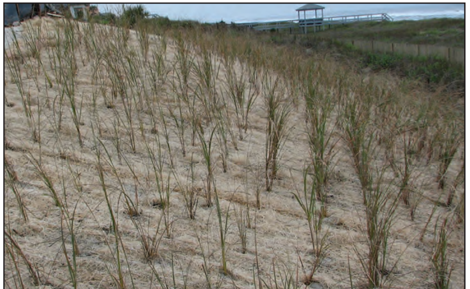
Innovation of netless products made plugging on slopes very easy. Photo courtesy of American Excelsior Company.
