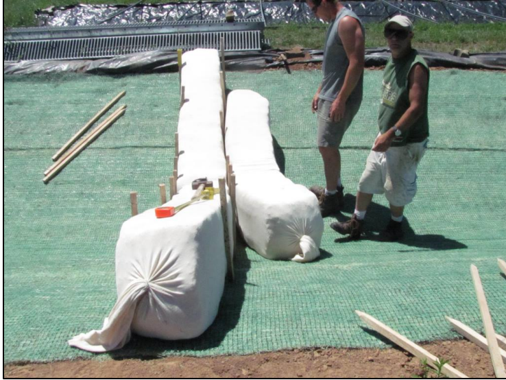
Figure 4. Installing second bottom row of Curlex Bloc filter station.
