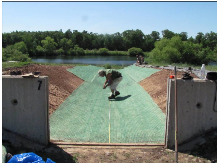
Figure 3. Installing Curlex Enforcer.
