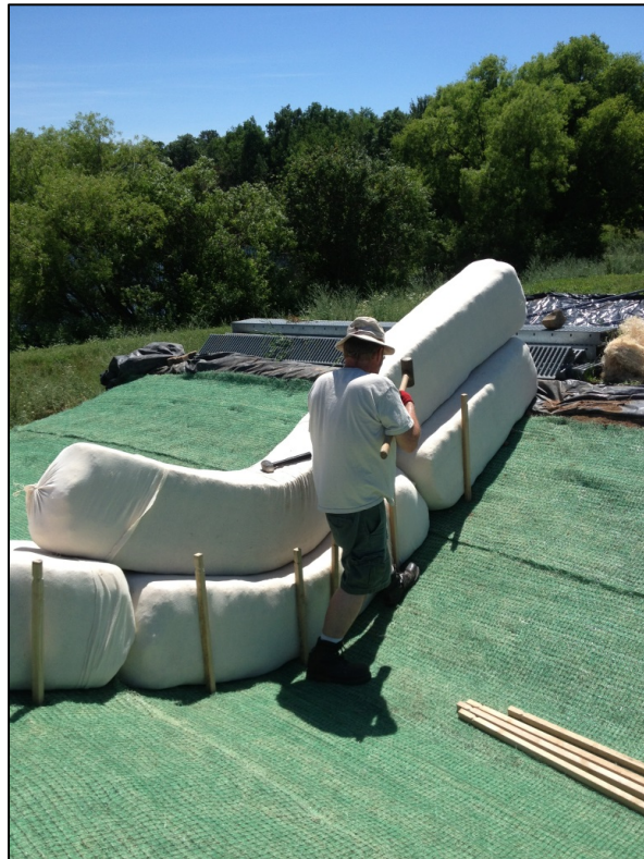
Figure 5. Pounding stakes for Curlex Bloc filter station.
