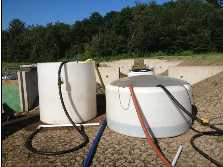
Figure 7. Tanks, pumps, and hoses before flow began.
