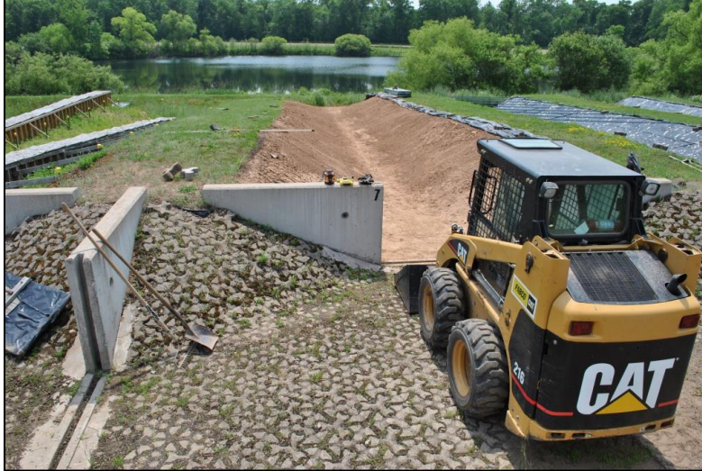
Figure 1. Prepared earthen channel before installation of Curlex Enforcer and Curlex Blocs.
