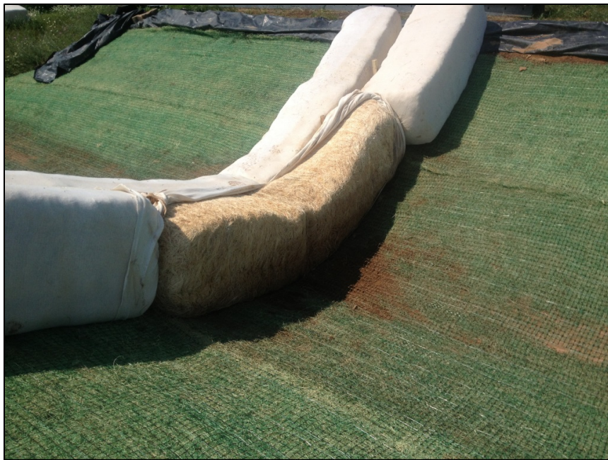
Figure 13. Containment material removed from front bottom Curlex Bloc after simulation.
