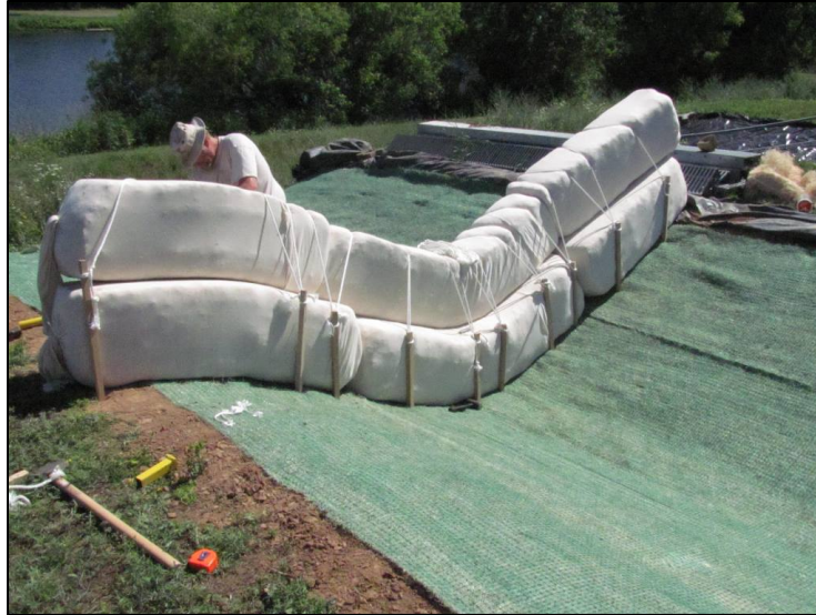
Figure 6. Wrapping rope to secure Curlex Bloc filter station.
