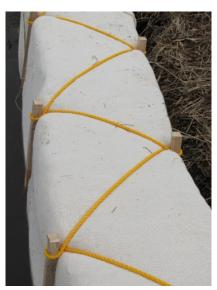
Step 5 Backfill to the top of the Curlex Blocs. If desired, seed and fertilize backfill area. Install  $\text{Curlex}^{\mathbb{R}}$  Netfree onto the backfill area. If desired, plug plants through the Curlex NetFree.
