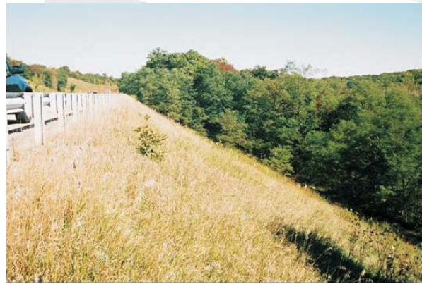
Figure 4. Figure 3 slope in 2004.
