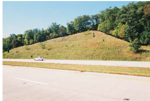
Figure 6. Figure 5 slope in 2004.
