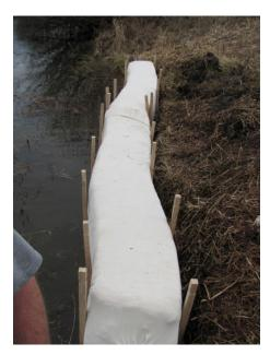
**Step 4** Weave rope from stake-to-stake, front-to-back along the length of the Blocs. Drive the stakes the remaining 3-4 inches or until the rope is tight.
