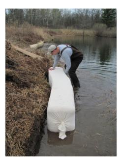
**Step 2** Place a second Bloc adjacent to the first Bloc. Pull the extra flap of containment material from the second Bloc over the end of the first Bloc. This will create a seamless joint between Blocs.
