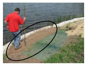
**Step 6** If desired, use a planting iron to create a pilot hole through the Bloc. Insert a live stake through the pilot hole into the subgrade a minimum of 6 inches below the Bloc.
