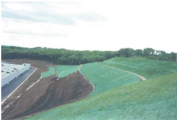
Figure 1. QuickGRASS® provides an instant finished look, while protecting steep, long slopes.
