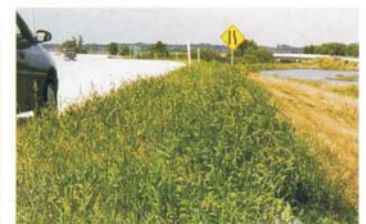
After Curlex I QuickGRASS installation, vegetation is established and the shoulder is protected.
