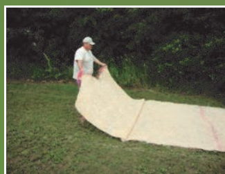
Figure 3. Walk ECB back, while holding near both corners.
