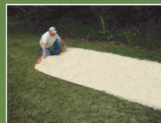
Figure 4. Properly position unrolled ECB for installation
