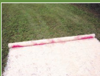
Figure 1. Locate red line near the end of the ECB.
