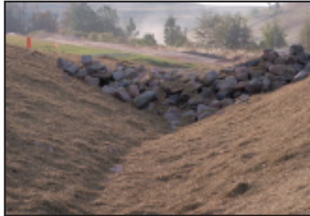
Rock check dam in ditch.
