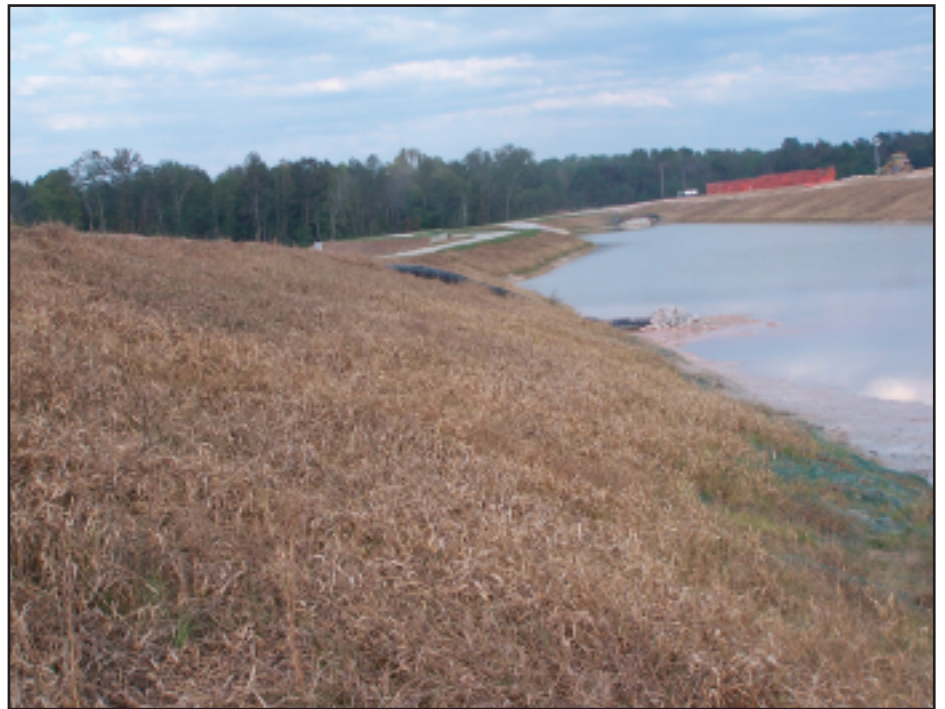
Vegetated side slope of stormwater pond.
