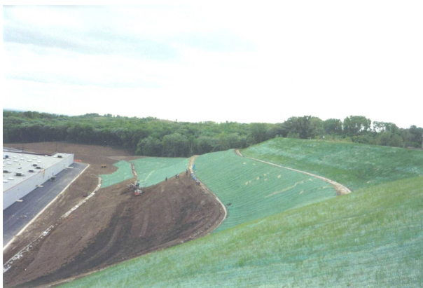
Figure 3. QuickGRASS provides an instant finished look, while protecting steep, long slopes.
