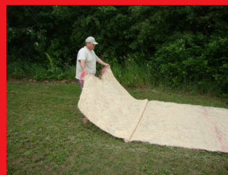
Walk ECB back, while holding near both corners.
