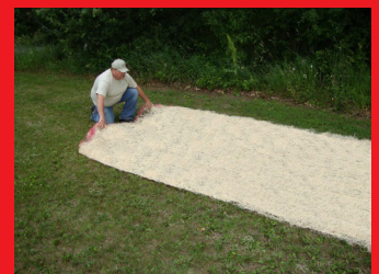
Properly position unrolled ECB for installation.
