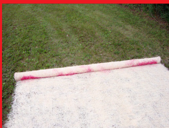
Locate red line near the end of the ECB.
