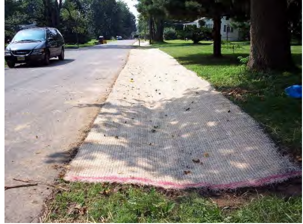
Curlex TRM Road Drainage After
