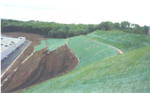
Curlex TRM During Installation
