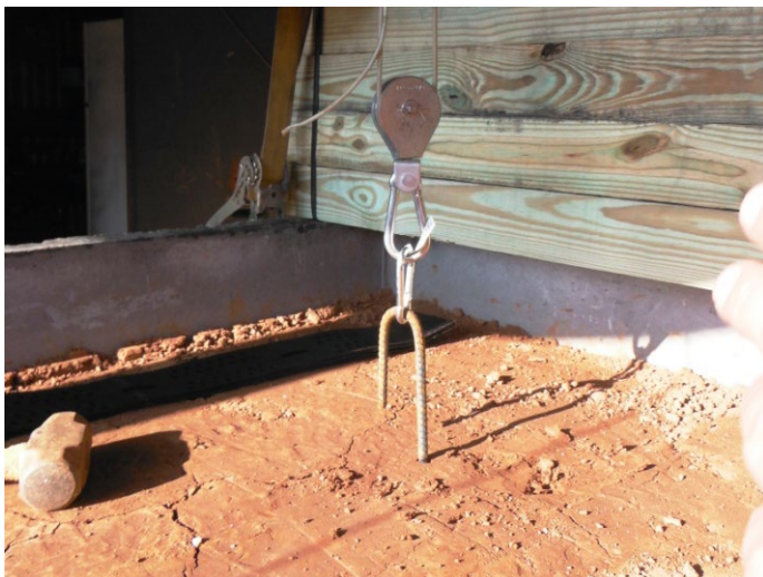
Figure 14: Pullout test of "J" hook in loam soil.
