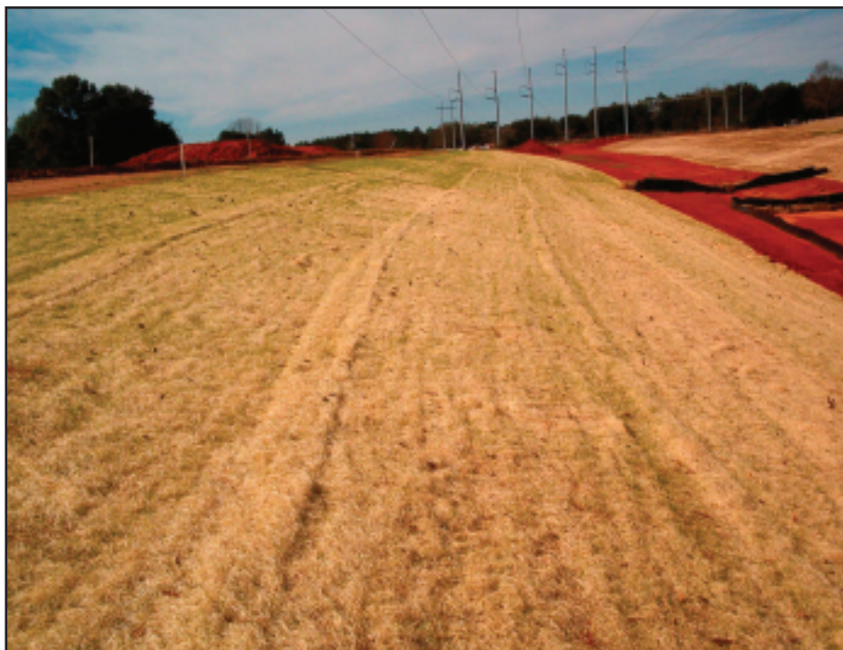
Net-less erosion control blanket protecting long stretch of golf course.
