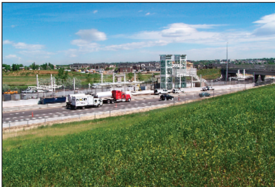
View of I-225 from top of completed berm.
