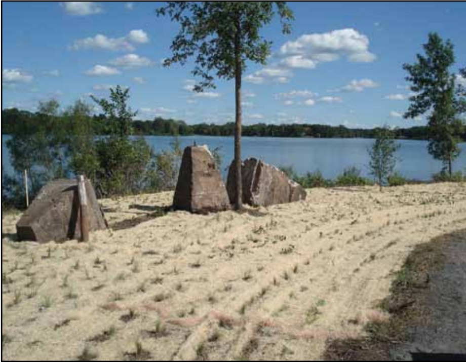
Native plugs through erosion control blanket on day of installation. Note Rice Lake in background.
