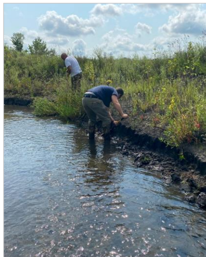
Figure 4: Streambank excavation and preparation.
