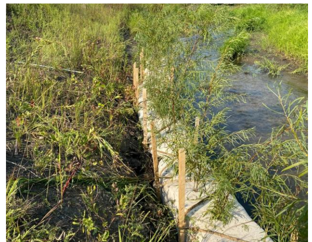
Figure 8: Curlex® Bloc with live stakes inserted.
