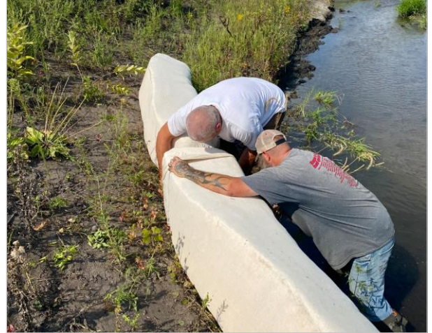
Figure 6: Fitting two Curlex® Blocs together.
