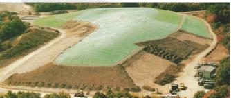
Approximately 77,460 yd<sup>2</sup> of QuickGRASS were used on the landfill project. Due to the large area to be covered, wide 8 ft rolls of Curlex blankets were chosen, to speed application time on the project.
