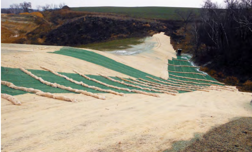
Curlex TRM Protecting Channel and Embankment
