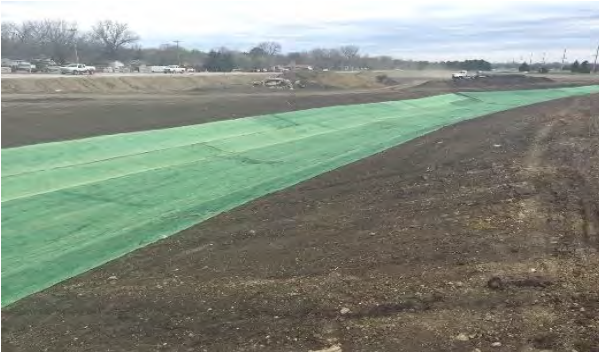
Curlex TRM Protecting Channel and Embankment
