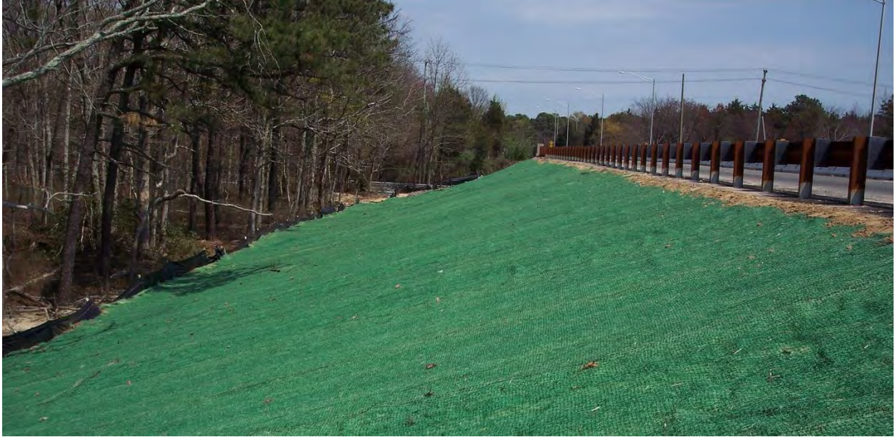
Curlex TRM on Roadside Slope
