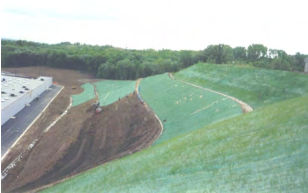
Curlex TRM During Installation
