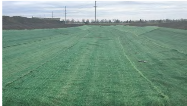
Curlex TRM Protecting Channel and Embankment
