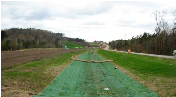
Curlex TRM Miles of Protection After Install
