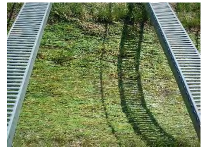
Curlex TRM After (No Soil Loss)
