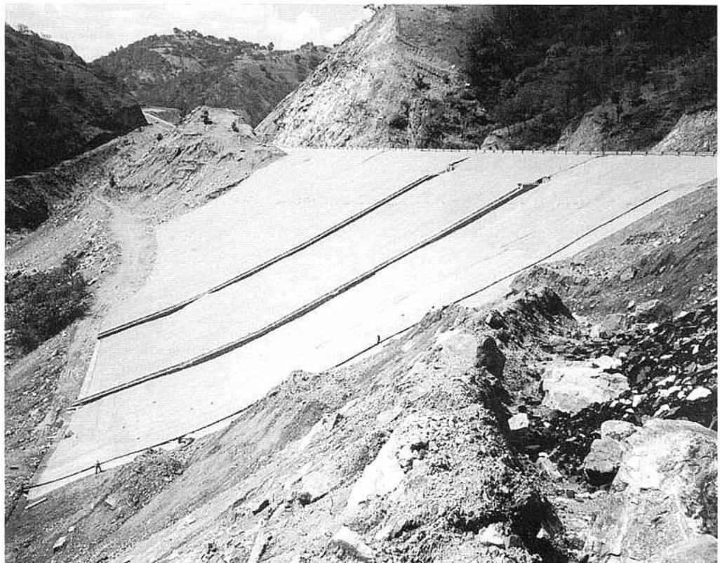
Photo 1. Green-dyed excelsior erosion control blanket protects 2H:1V slope along the Autopista north of Oaxaca, Mexico.
