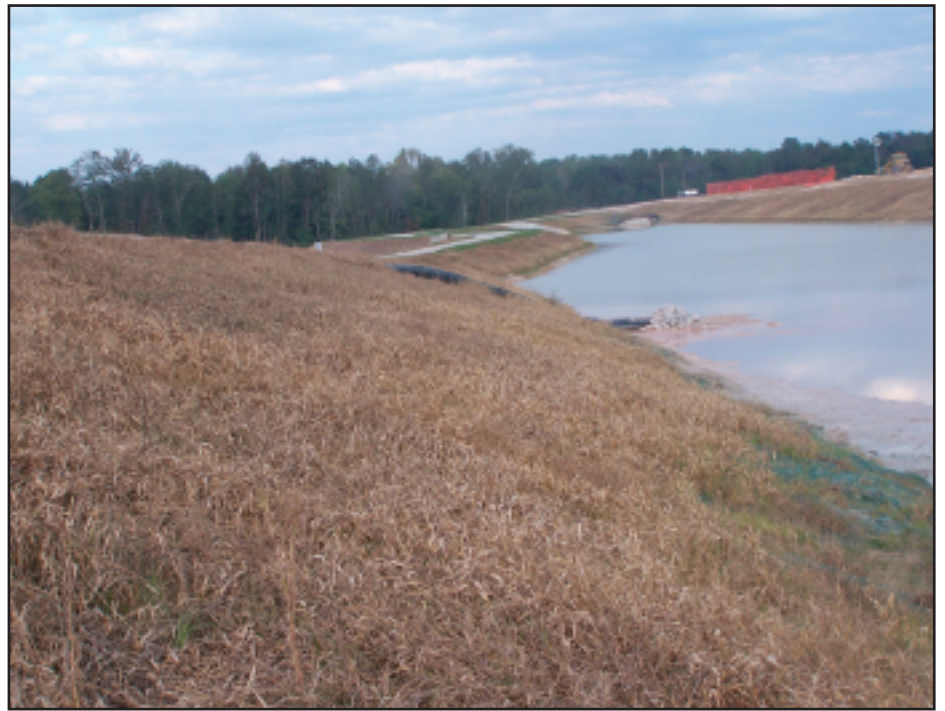
Vegetated side slope of stormwater pond.
