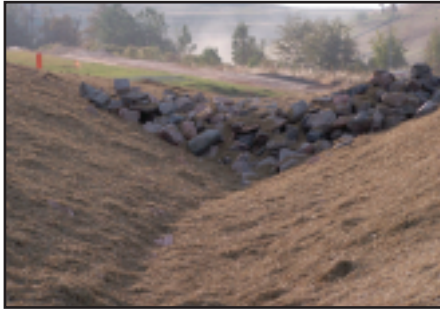
Rock check dam in ditch.
