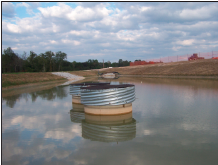
Top: Landfill expansion continues behind stormwater ponds. Below: Overflow structures in stormwater pond.
