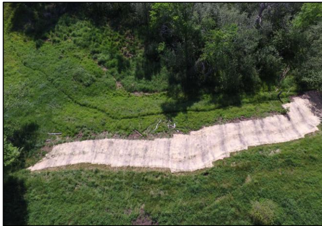
Figure 5: Aerial view of completed Curlex II spring installation.
