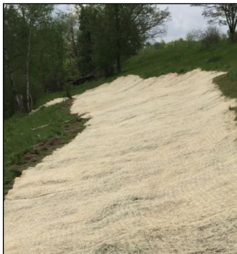
Figure 4: Completed installation of Curlex® II on the disturbed slope.
