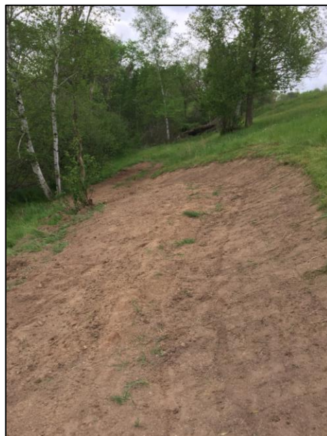
Figure 3: The exposed area after clearing, raking, compacting, and seeding.
