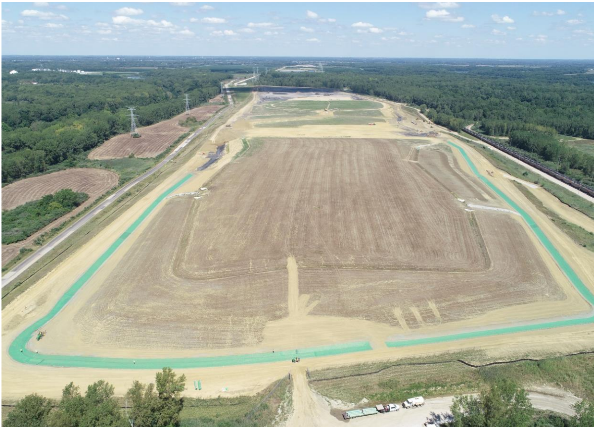
Figure 6. Recyflex TRM-V Installation Around Pond Perimeter
