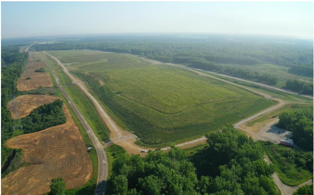
Figure 7. No Erosion on Pond Where Recyclex TRM-V was Installed
