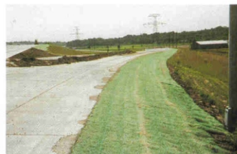
Curlex I QuickGRASS protects the shoulders from stormwater runoff before vegetation is established.
