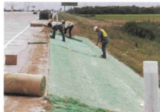
Using 8 ft. wide rolls enable Curlex I QuickGRASS installation to progress quickly and easily.
