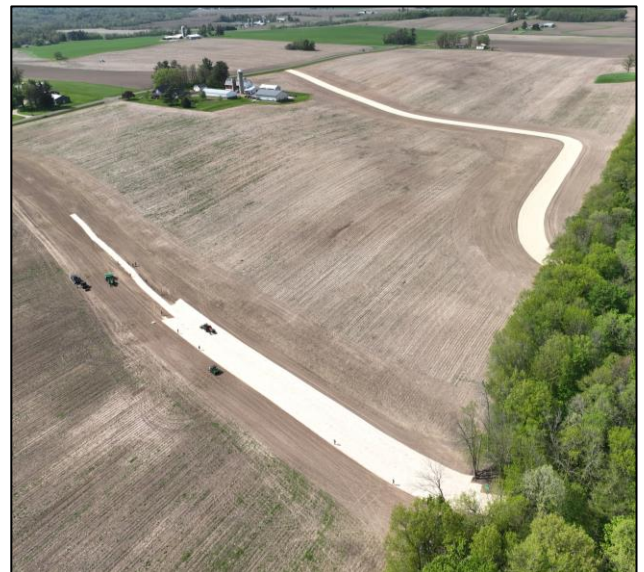
Figure 5: Curlex II ECBs being installed in 8' widths to cover each swale.
