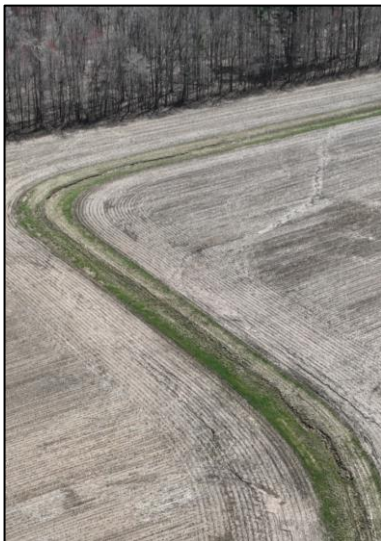
Figure 1: Aerial view of one swale on the property before excavation. Notice the large gully running down the middle of the swale from years of erosion.
