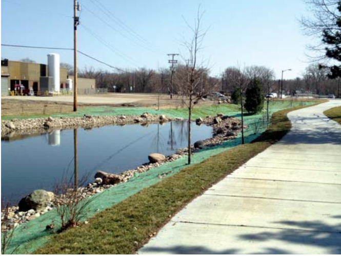
Sediment pond lined with TRM (March 2012).
