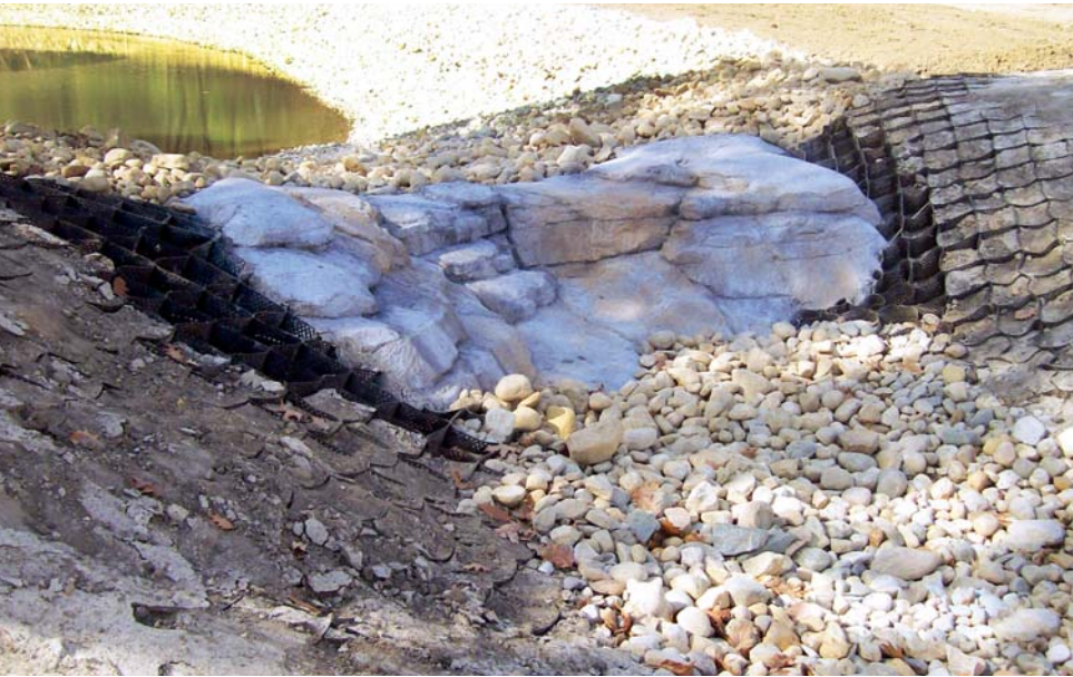
Concrete/decorative clad drop structure installation at sediment pond outlet (October 2011).
