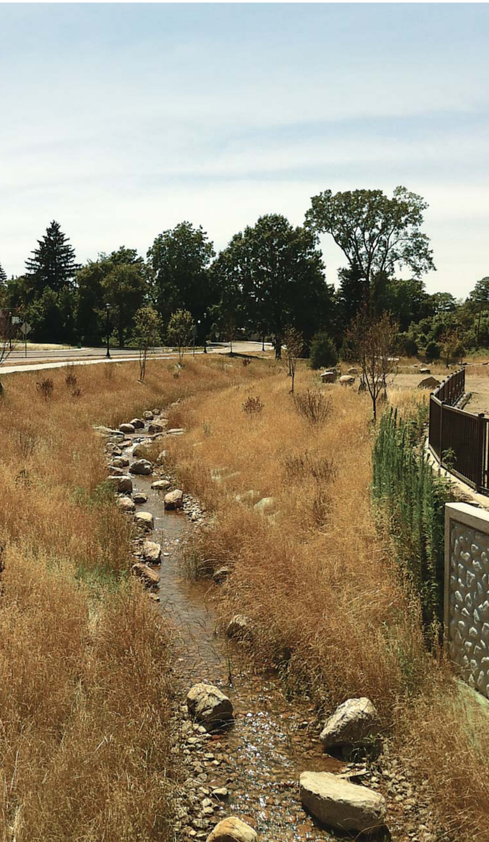
Channel upstream of intersection (June 2012).
