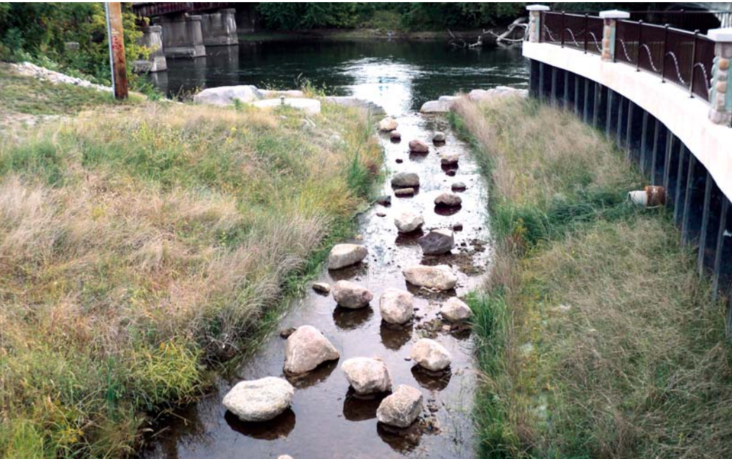
Stormwater channel outlet to the St. Joseph River (September 2012).
