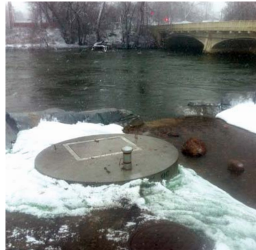
Stormwater channel outlet to St. Joseph River (January 2012).
