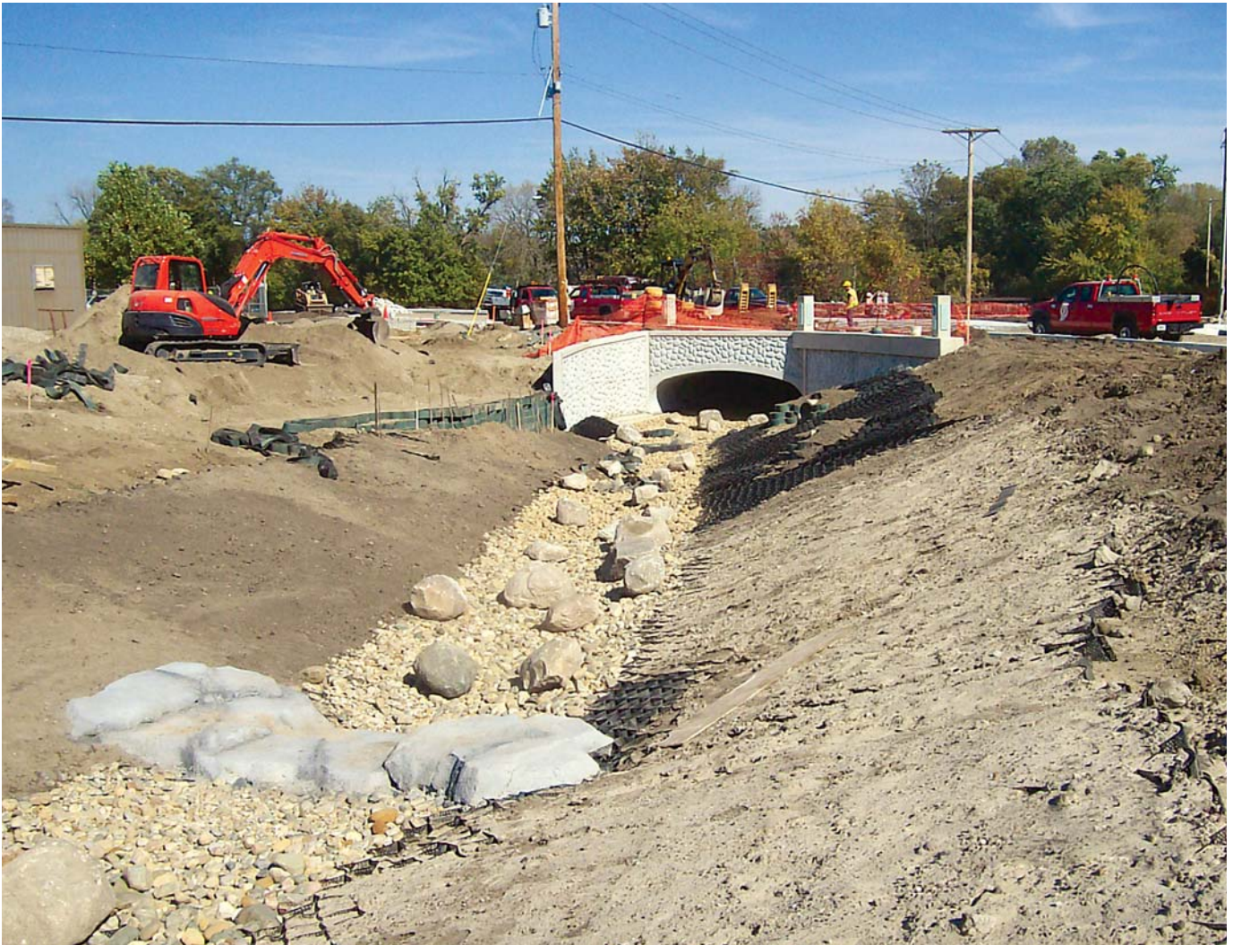
Channel construction before the turf reinforcement mat (TRM) was installed (October 2011).
