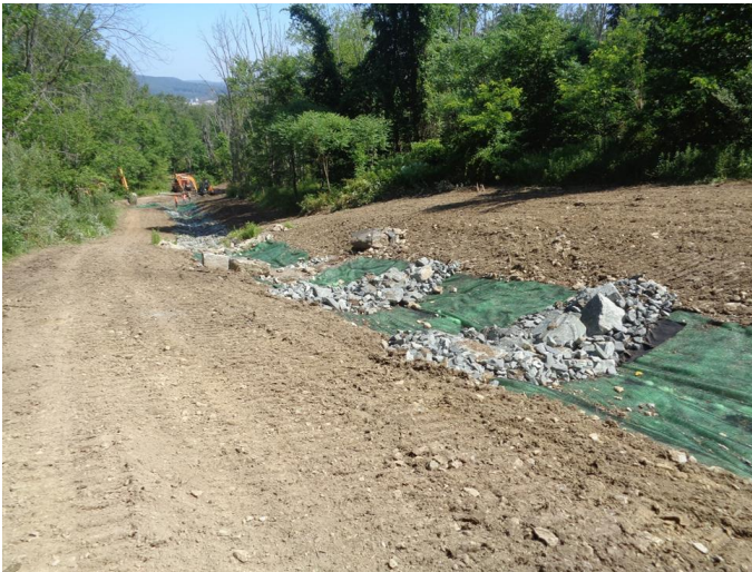
Figure 8. TriNet Recyclex and New Rock Check Dams
