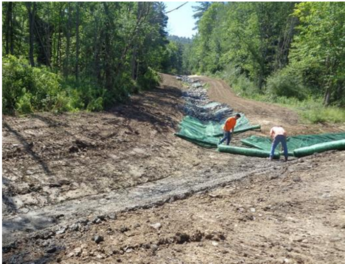
Figure 6. Installation of TriNet Recyclex
