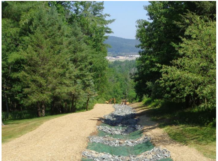
Figure 9. AEC Premier Straw Installed Outside Channel
