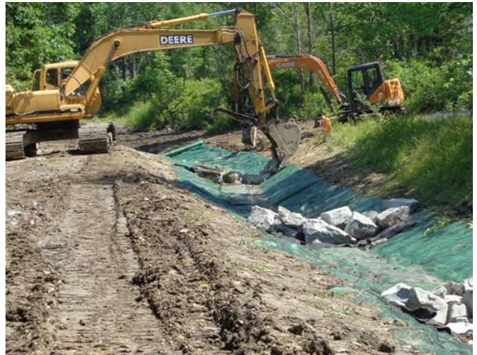
Figure 7. New Rock Check Dams Over TriNet Recyclex
