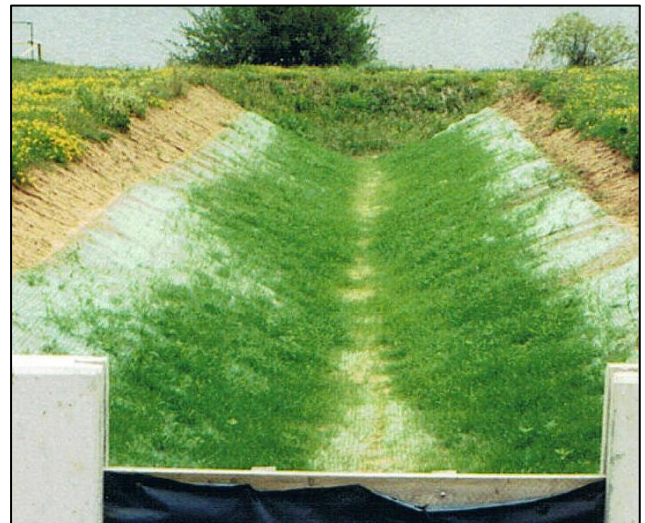
Figure 6: Recyclex TRM installation results after 33 days.
