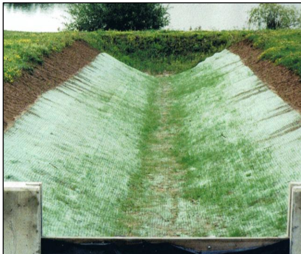
Figure 5: Recyclex TRM installation results after 22 days.
