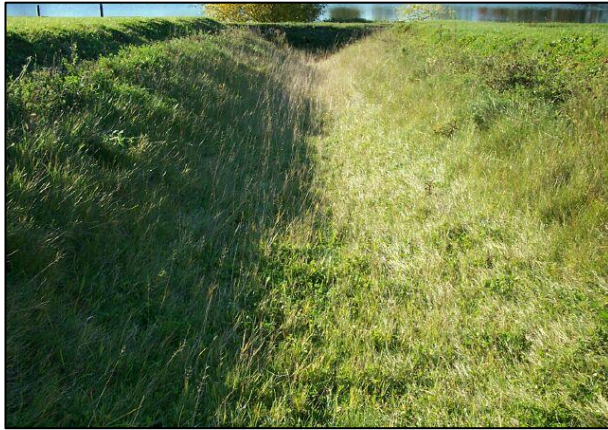
Figure 7: Recycllex TRM installation results after 2 years.
