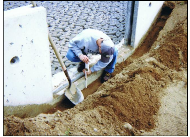
Figure 4: Digging a trench in which to install the Recyclex TRM at the head of the channel.
