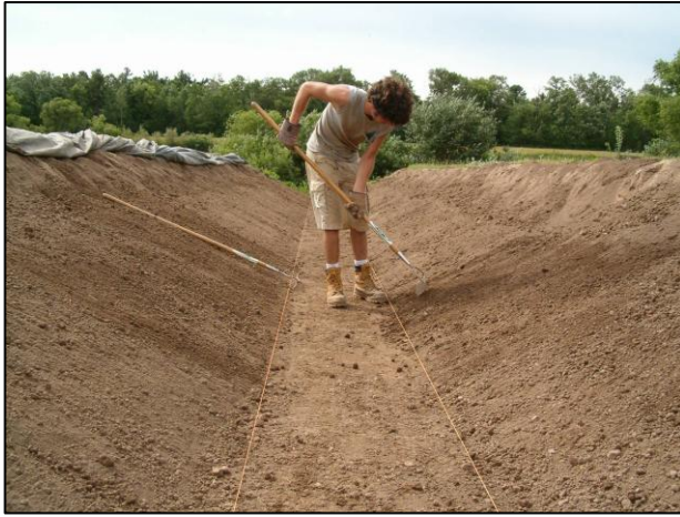
Figure 3: Example of removing roots and rocks from the subgrade.
