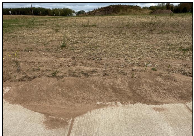
Figure 2. Failed blown straw installation that led to sediment being deposited onto the sidewalk.
