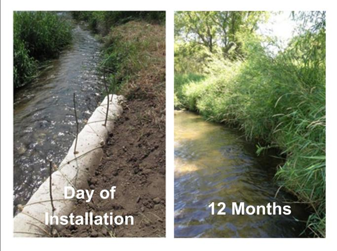
Curlex Blocs are suitable for streambank restorations and other shoreline applications with low energy and wave action. In this installation, willow live stakes and native sod were used to restore and protect this site.
