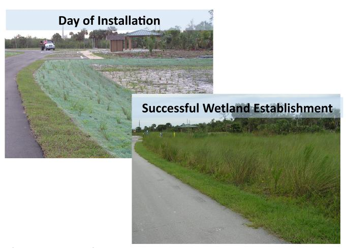
Curlex I Erosion Control Blankets provided the protection required for this sensitive wetland. Proven Curlex fibers protected the sandy seed bed and ensured optimal growing conditions in extremely challenging climatic conditions.
