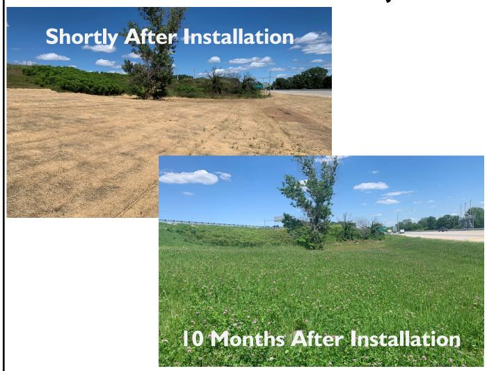
Curlex<sup>®</sup> II FibreNet<sup>™</sup> was the natural choice for this roadside project. Proven Curlex Aspen excelsior fibers and two layers of FibreNet jute netting combine to create a blanket designed for slopes up to 1.5H:1Vs and for channel flows up to 9.0 ft/s (2.7 m/s) and 2.25 lb/ft² (108 Pa) shear stress.
