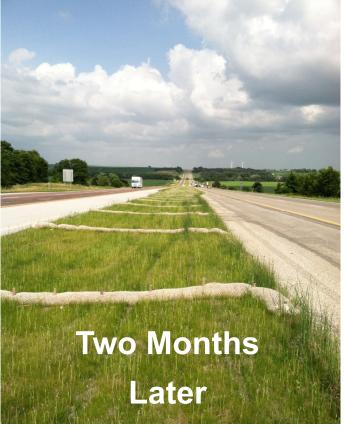
Curlex Sediment Logs were chosen for this environmentally sensitive highway project. Porous Curlex Sediment Logs are engineered to both dissipate velocity and filter contaminated runoff before it discharges to precious water resources. Curlex Sediment Logs were installed along with Curlex erosion control blankets on this project. Both of these excelsior based products are made from sustainably harvested Great Lakes Aspen and are naturally seed free.
