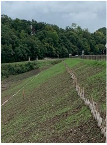
Curlex<sup>®</sup> Sediment Logs protected this steep, unprotected dam during early stages of construction. During rainfall events, the Curlex Sediment Logs slowed sheet flows and captured sediment both within the Curlex<sup>®</sup> fibers and up slope of the logs themselves. All of these features resulted in good establishment of the temporary vegetation and kept the site in very good shape until the site was ready for final grading and seeding.
