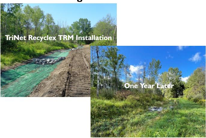
The Recyclex® family of TRMs have been protecting our natural resources for over 20 years! They are made using recycled post consumer waste fibers. Unlike other many other TRMs, TriNet Recyclex® does not float. This ensures good contact with the soil during hydraulic events. TriNet Recyclex® does not inhibit vegetating growth. In fact, the light color can help prevent seed burnout.
