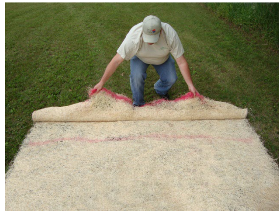
Figure 2. Pull end of RECP along red line.
