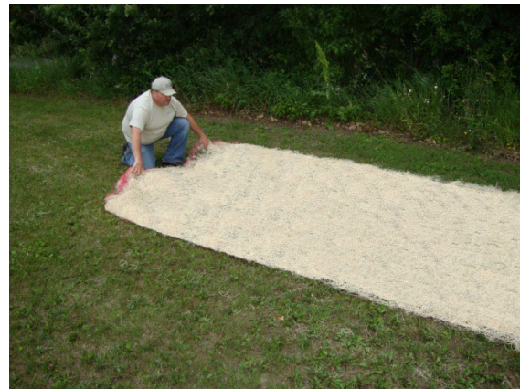
Figure 4. Properly position unrolled RECP for installation.
