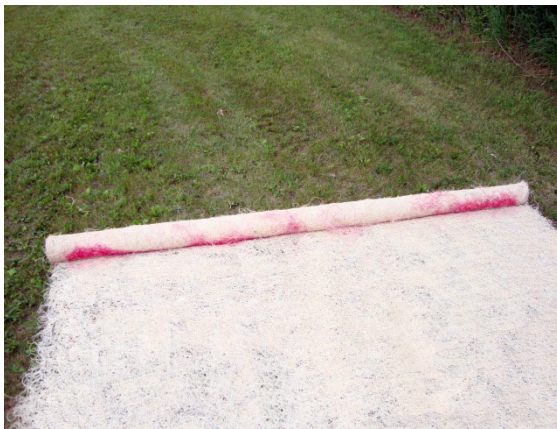
Figure 1. Locate red line near the end of the RECP.
