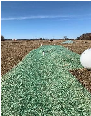
Curlex Septic Blanket Installed.
