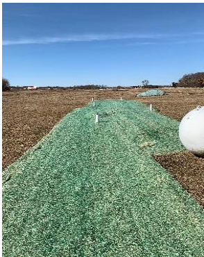
Curlex Septic Blanket Installed.
