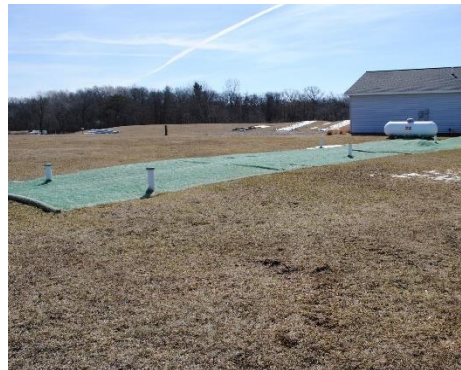
Curlex Septic Blanket Installed across drain field before significant snow cover.
