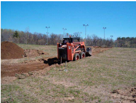
Figure 2. Removal of sod and existing topsoil.
