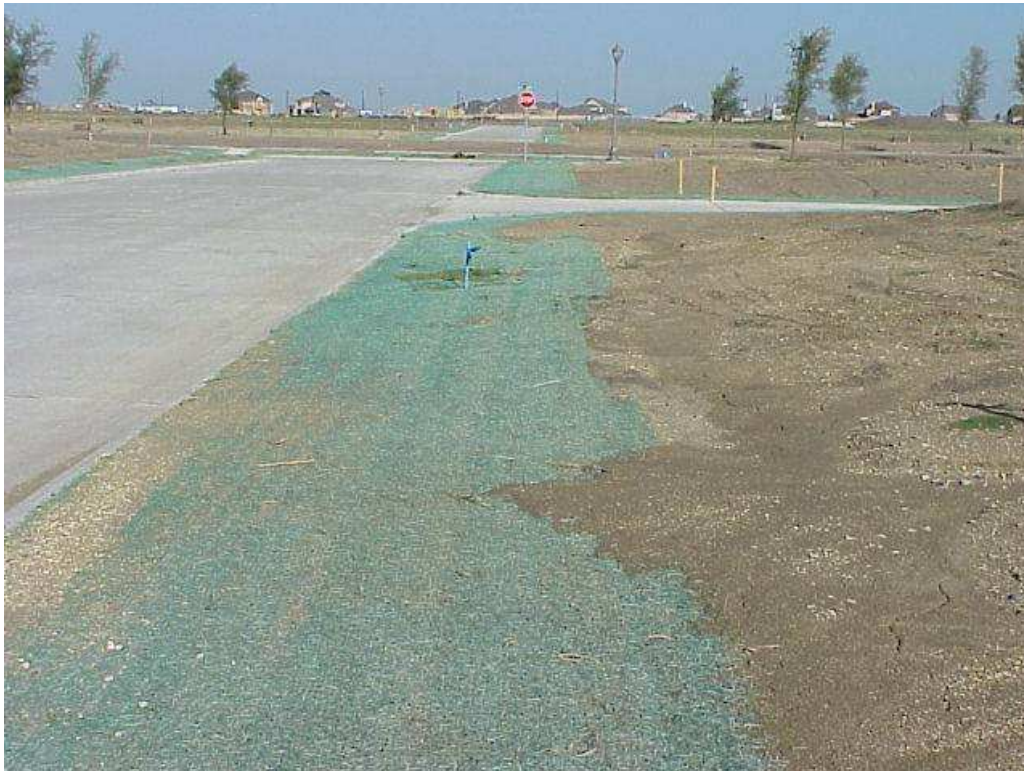
Figure 1. Excelsior buffer strip used for perimeter erosion control.
