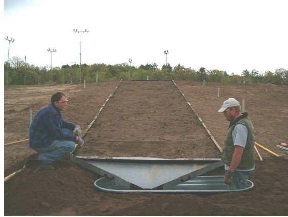
Figure 7. Completed plot with collection tank buried at the toe.
