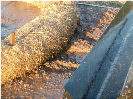
Figure 7. Rill under 30.5 cm straw wattle during 10.2 cm/hr segment.
