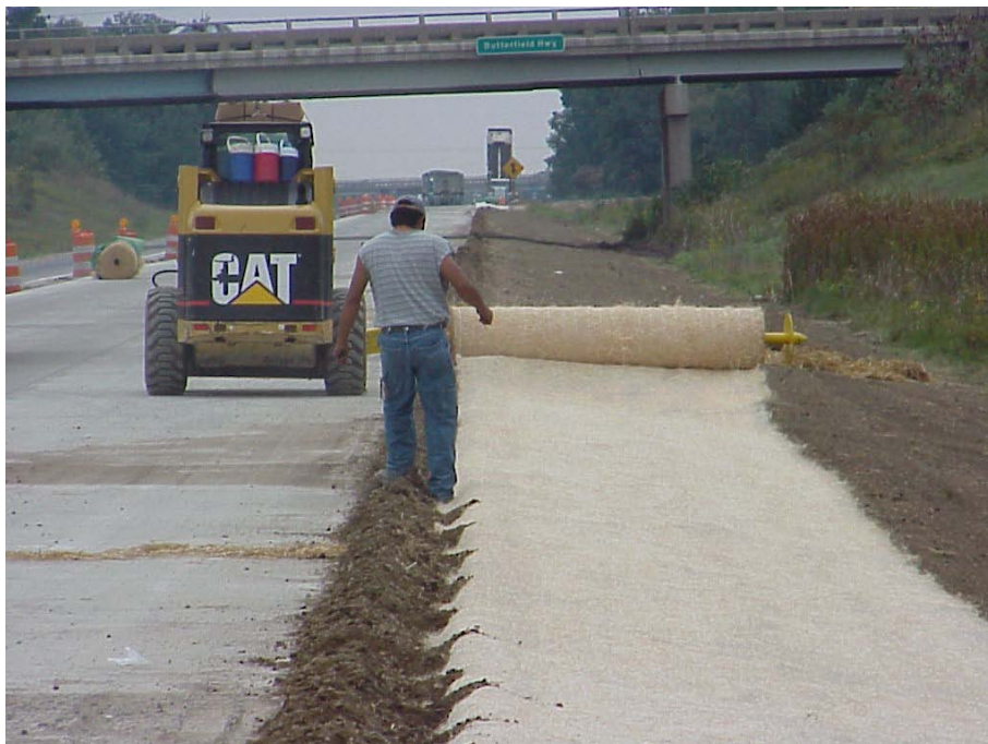
Figure 12. Mechanical installation of Curlex RoadRunner.
