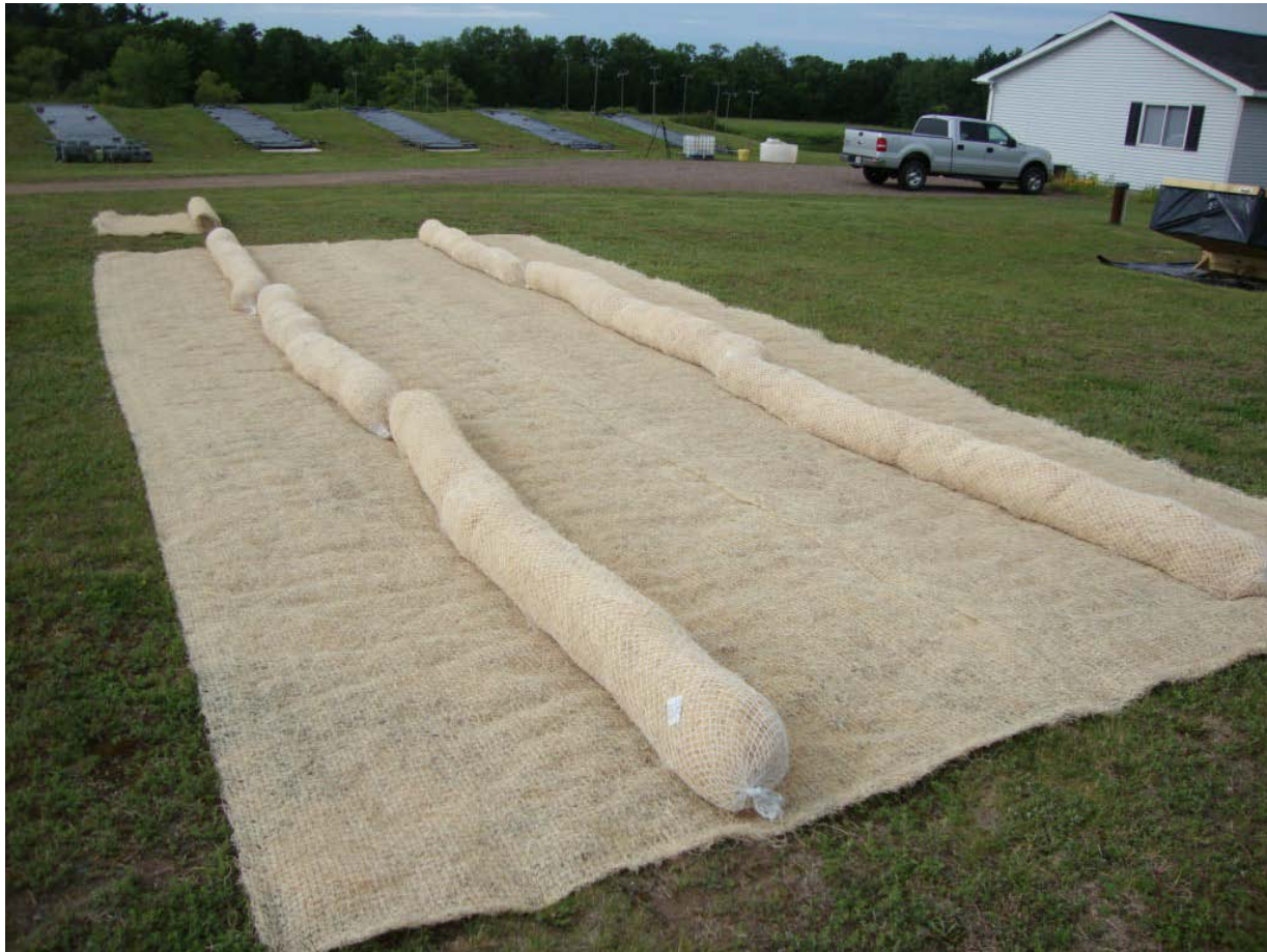
Figure 10. Curlex blankets (16' wide of Curlex fibers stitched between two layers of netting shown) with Curlex Sediment Logs (Curlex fibers encased in tubular netting) on top. Note in the upper left of the photo a "roll" of Curlex. Photo taken at ErosionLab®, which is owned and operated by American Excelsior Company. ErosionLab is the largest privately owned testing laboratory of its type.
