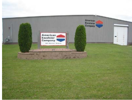
Figure 17. View from Pioneer Avenue.
