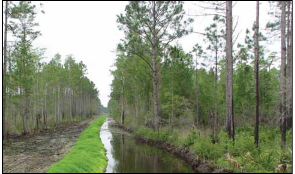
Vegetated erosion control blankets protecting bank a few weeks after installation (left side of photo).
