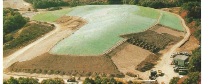
Approximately 77,460 yd<sup>2</sup> of QuickGRASS were used on the landfill project. Due to the large area to be covered, wide 8 ft rolls of Curlex blankets were chosen, to speed application time on the project.
